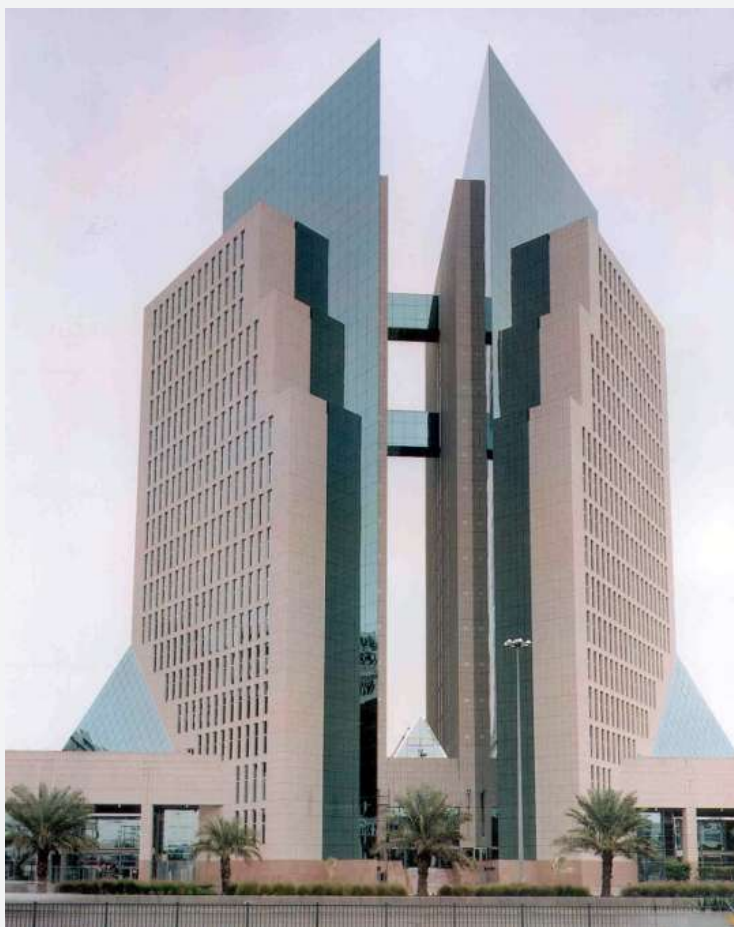
First headquarters of the Capital Market Authority, Tawuniya tower, Riyadh (2003).
